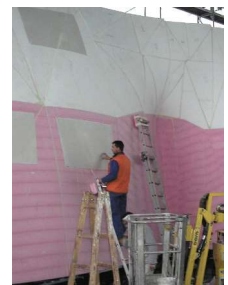
Application on a polystyrene foam or other type support
