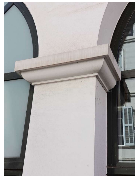
Detail of a column cladding on the facade of the Majestic Hotel – Cannes - Acrystal Prima + Acrystal 200-4D fiber - Laminated panels +/- 7 mm thick
